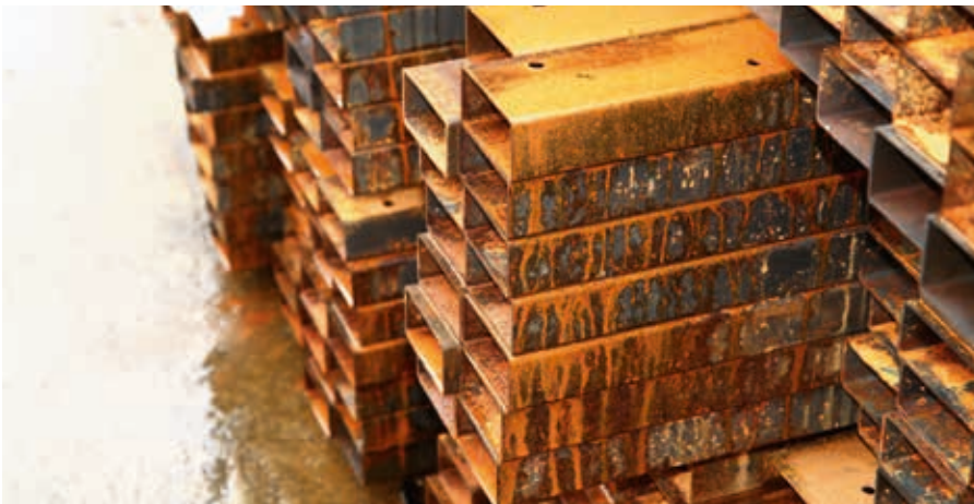
Fig. 4: Corrosion of steel components.
