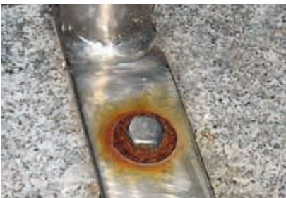
Fig. 12: This is a typical case of contact corrosion. Zinc-plated carbon steel (washer) and stainless steel (screw and part) were used together. The surface area of the more noble metal – the stainless steel – is larger, causing strong corrosion of the washer.
