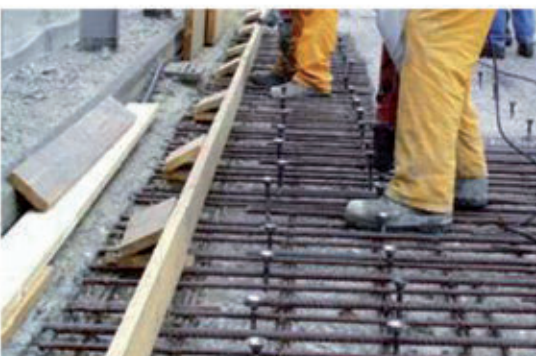
Slab strengthening
