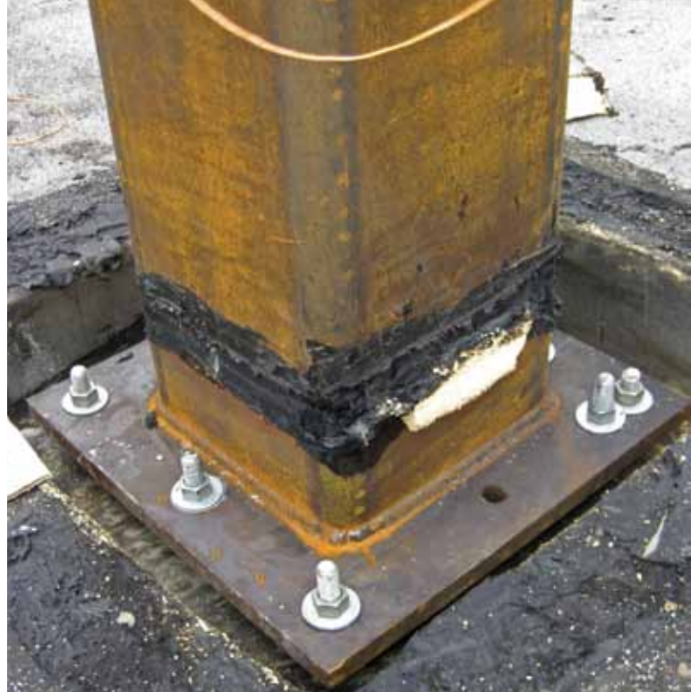
Fig. 4: Details must set limits on how anchor locations are adjusted. In this installation, a second borehole (as well as a new hole in the base plate) had to be drilled because the drill bit contacted a reinforcing bar at the original location. The anchorage capacity will be reduced, however, because the resulting anchor spacing is too small
