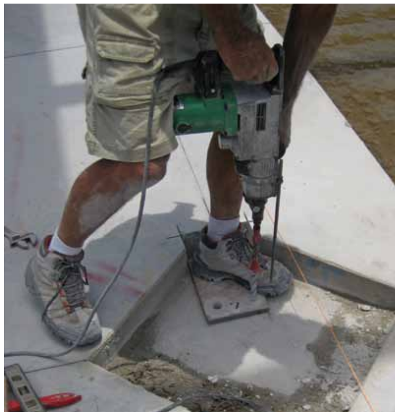
Fig. 6: The correct method for creating a borehole. The installer is drilling through a template using a hammer drill with a depth stop
