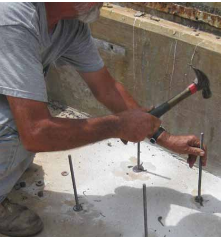
Fig. 5: After the boreholes were filled with adhesive, these threaded rods were hammered into place because the hole was too small. The size of the drill bit required for a given anchor diameter should be clearly communicated in the MPIs
