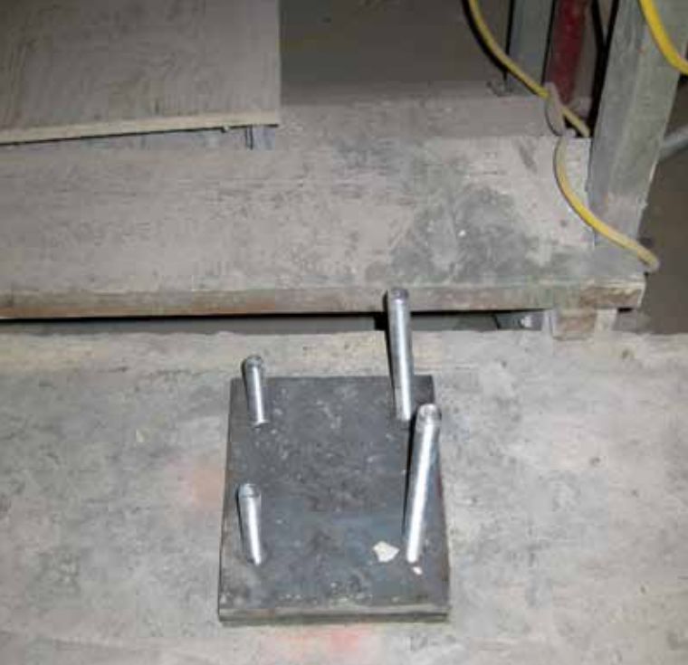
Fig. 3: To avoid interference problems, reinforcing bars must be located before drilling and provisions must be made in the details to allow adjustment of anchor locations. Otherwise, bars would be drilled through reinforcement and affect the capacity of the structure. Here, the installer attempted to clear initially undetected bars by inclining the boreholes. The long extensions on two of the threaded rods show that the attempt was a failure
